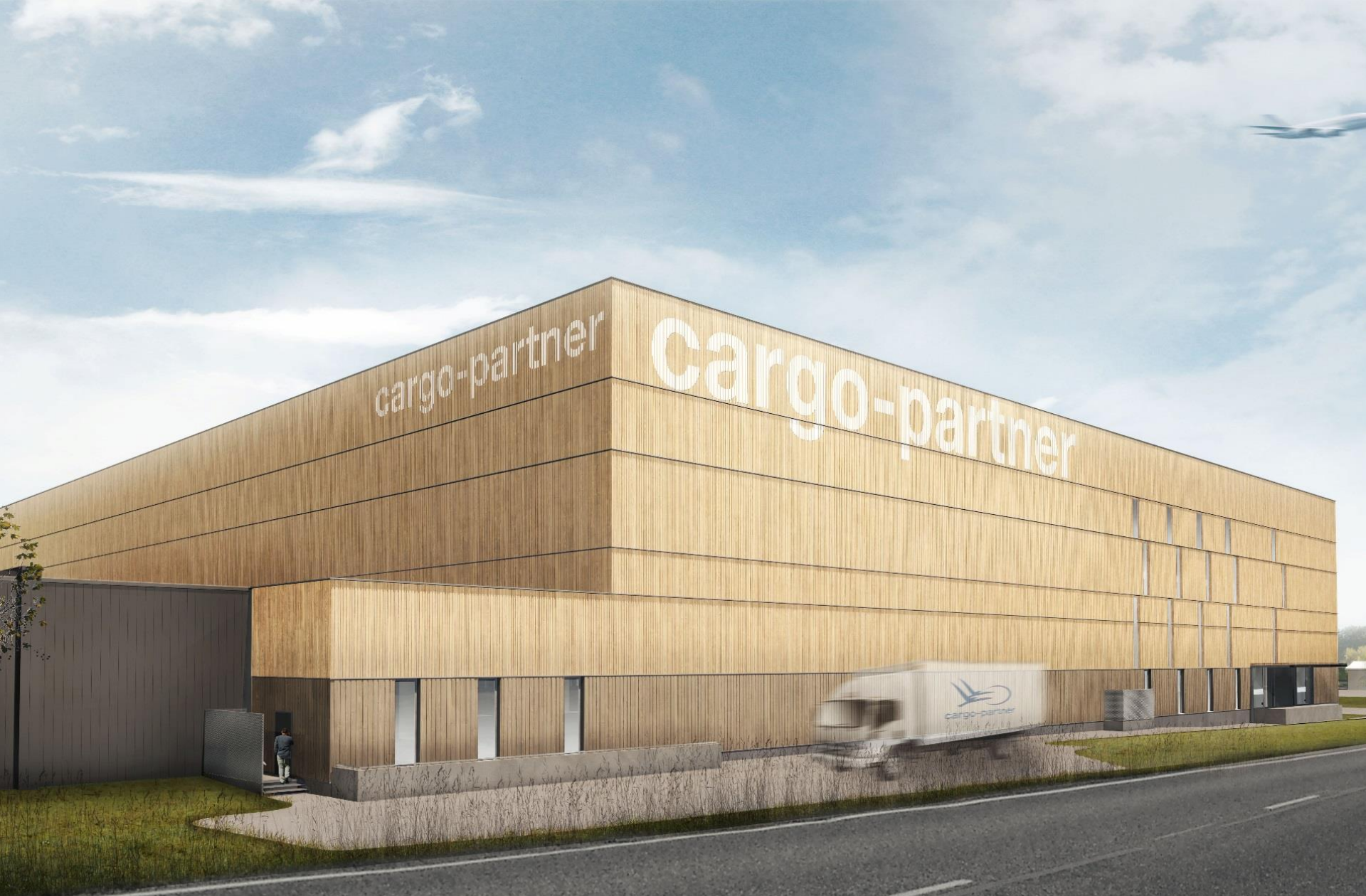
Cargo Partner logistic hall, Fischamend hall completely made out of timber, 4.300 m3 used timber Poppe * Prehal Architects
