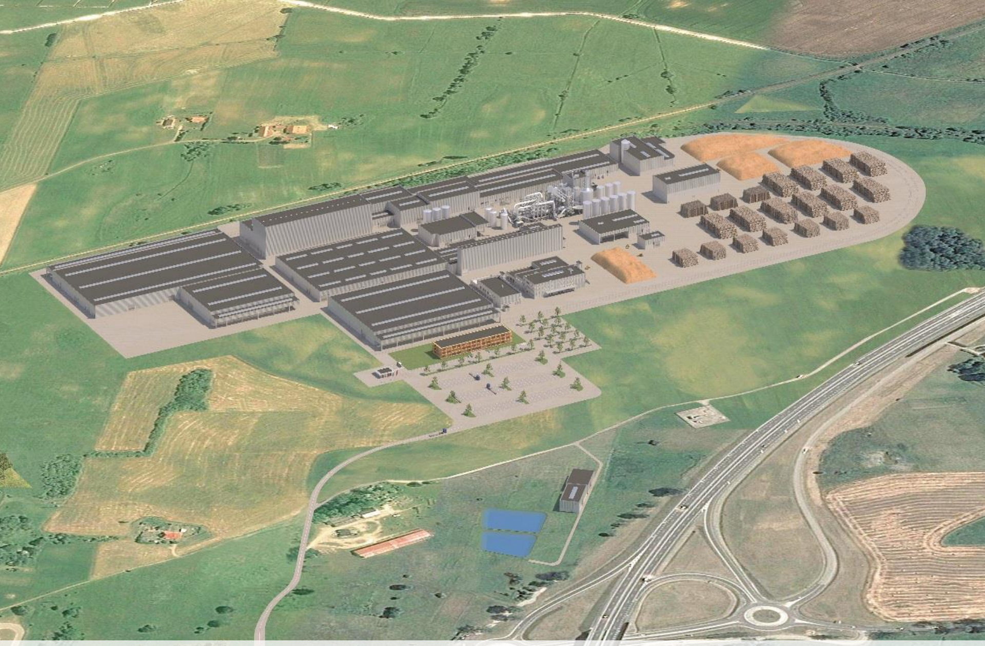
Production plant Egger, Polen
